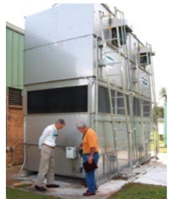
Tank Motes and Sherman Phillips look at the cooling tower that was installed last summer at Ochwilla Elementary School. In conjunction with the tower, frequency drivers allow for the lowering of water flow during times when air conditioning is not needed. These upgrades allow for better cooling and efficiency.
