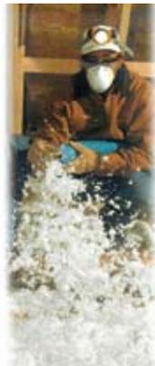
Typical bulk insulation products, such as blow-in fibers, can qualify for the tax credit. The tax credit does not include installation.
