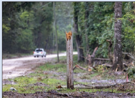
A broken pole in the Lake City District, one of the areas most impacted by Helene.
