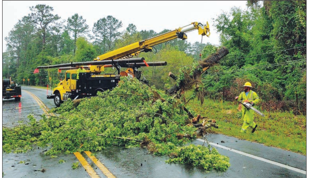
Crews work as quickly and safely as possible to restore service after an outage.
